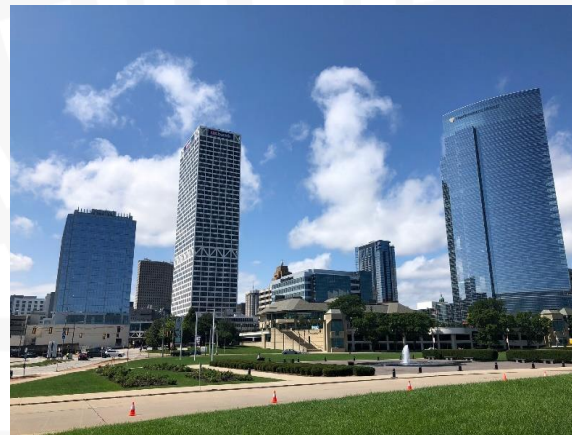
833 East & Northwestern Mutual's headquarters are two of several new developments near the lakefront in the Central Business District
