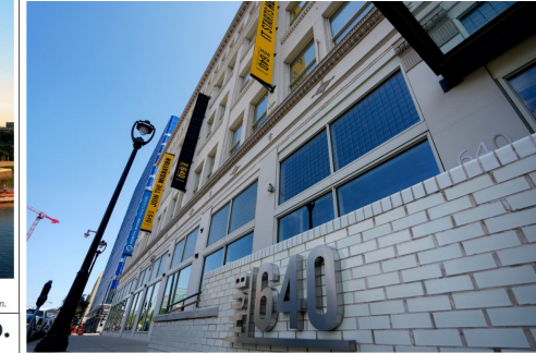
Fiserv will lease around 160,000 square feet at HUB640, the redeveloped former Boston Store building on N. Phillips Ave. Ebony Cox / Milwaukee Journal Sentinel
