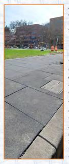
Just before winter, construction crews were able to complete the underground wiring, new water and sewer service on Wells Street, street light removal and re-installation, the new curbing, repairing the street pavement, ADA corner ramps, tree wells, sidewalk foundation slabs and a rough grading of the adjacent lawn. A partial install of the pavers was also completed as part of Phase 1 of the project.
